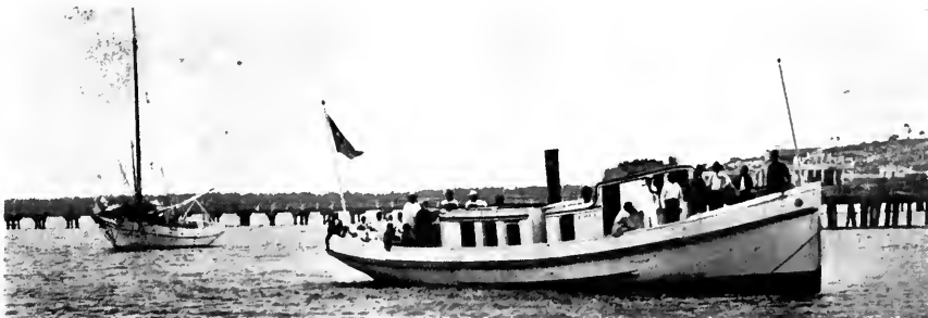
Tug "Juba," of the Atlantic Fruit Company, equipped with a 70-hp. four-cylinder Fulton Diesel engine.
